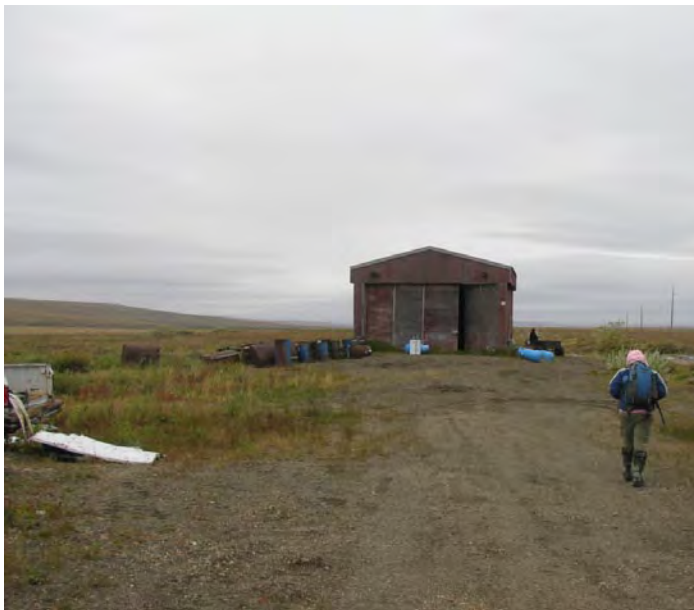
Figure 12. City-owned garage with 55-gallon drums and dump debris. (©TNSDS)
