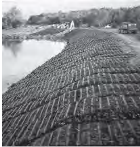
Figure 24. Example of a marine mattress used for erosion protection (Photo source: tensor.com)
