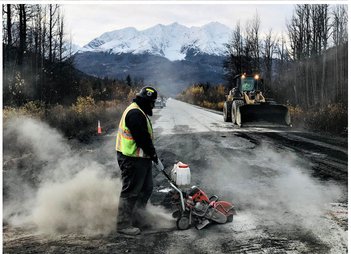
Saw cutting, Richardson Highway project. By Benoit Pignon, Alaska DOT&PF
